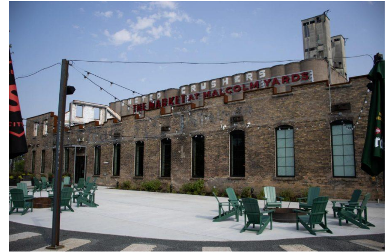
The Market at Malcolm Yards, 501 30 th Avenue S 13,000 square feet
