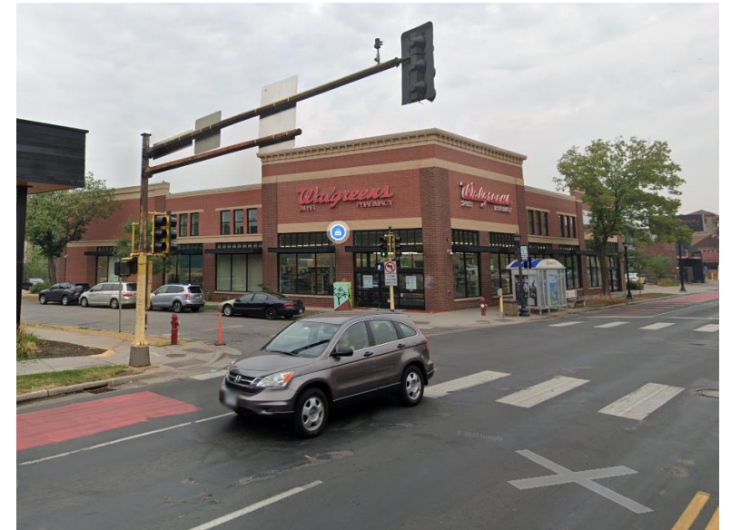
Walgreens, 2650 Hennepin 16,000 square feet
