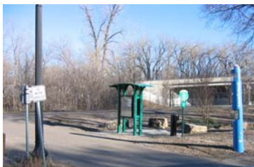
Access to the Greenway is obtained at grade (above) or via ramps or stairs.
