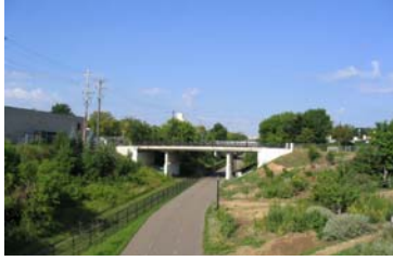
Midtown Greenway at Lyndale Avenue (Soo Line Gardens at right)
