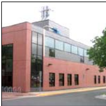
It is typical for institutional buildings to be oriented inward and away from Riverside Avenue.
