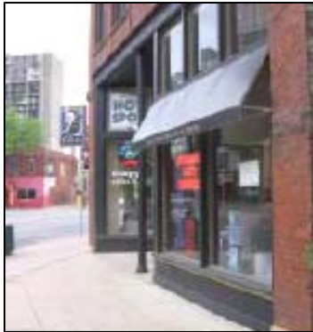
Traditional shop fronts orient display windows and entries to the street and sidewalk.
