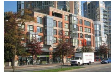
roof terraces and podium
