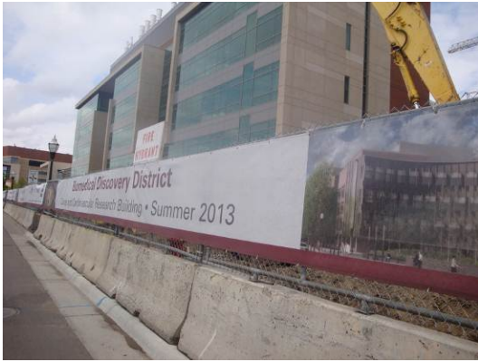
New University research building under construction
