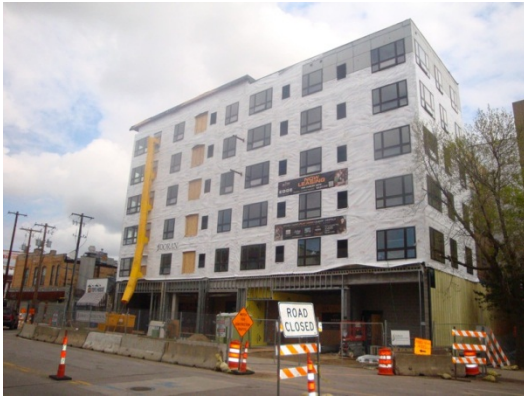
Student housing project under construction
