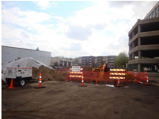
Light rail construction at Prospect Park station area
