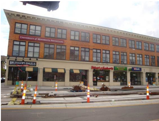
Stadium Village business access is being impacted by light rail
