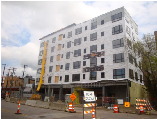
New student housing under construction
