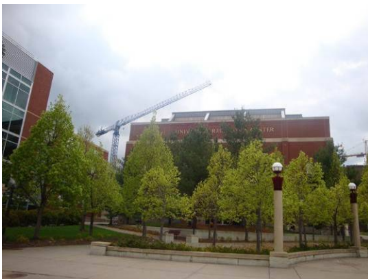
Building construction underway on University campus
