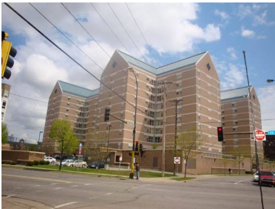
Student housing near Stadium Village
