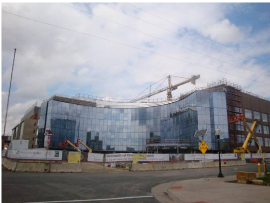
New University research facility under construction
