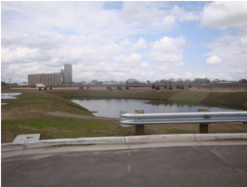
New stormwater pond in industrial area
