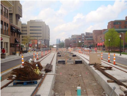
Central Corridor under construction through campus
