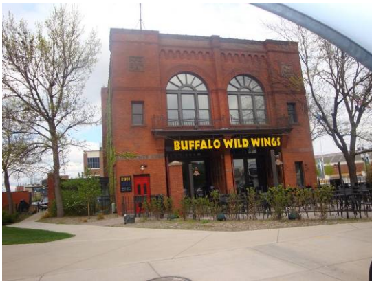
Renovated Fire Station #19 building
