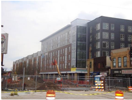
New housing under construction
