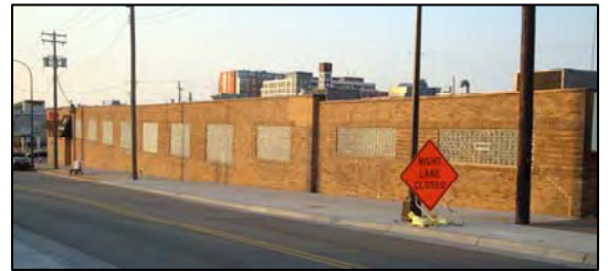
Figure 6.21 Example of poor street frontage
