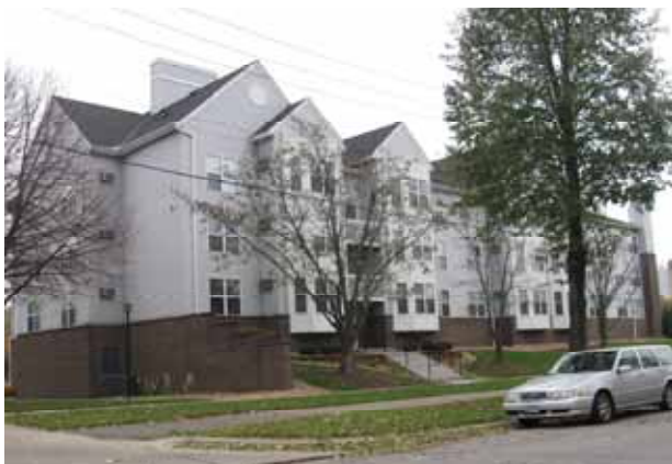
Recently constructed townhomes along 3rd Avenue.
