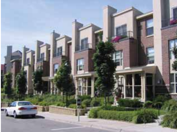
Attached, medium density row housing recommended for the area south of 3rd Avenue in proximity to a future Nicollet-Central modern streetcar station.
