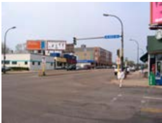
Existing road conditions at 54 th and Lyndale make pedestrian crossing difficult
