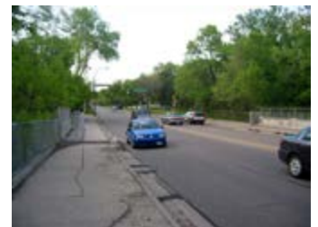
Reconstruction efforts at the Minnehaha Creek Bridge should focus on creating a more pedestrian-friendly and identifiable bridge into the district
