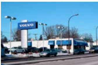
Several auto-oriented uses exist in the corridor
