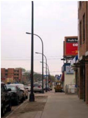
Existing streetscape conditions along Lyndale Avenue near 54 th Street
