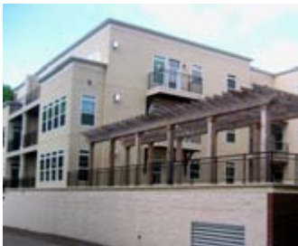
Buildings should be massed to reduce bulk near the top, to the rear of the building and should complement structures surrounding them
