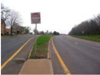
State Highway 121 is not designed to encourage pedestrian use.
