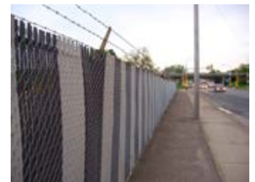
Existing fencing along Centerpoint Energy site faces Lyndale Avenue
