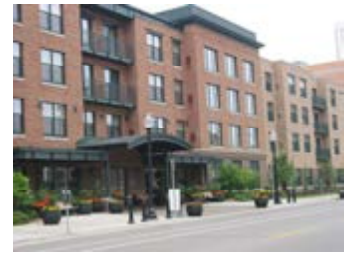
Changes in the massing of street-oriented building facades should include variations in wall plane and building height and reflect the dimension of building uses, residential units, room sizes or structural modules
