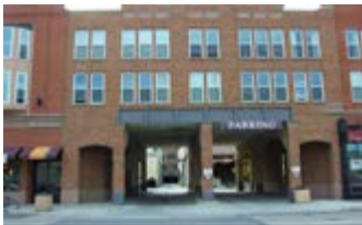
Conceal view of parking structures
