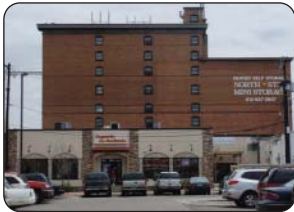
An example of a well-maintained restaurant in the foreground and in the background, a 9-story warehouse that should remain.
