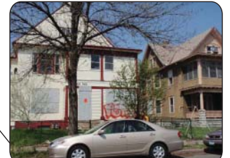
Many residential structures on Chicago Ave are currently vacant, boarded, and in some cases, condemned. In 2009, there will be a Chicago Avenue corridor planning effort led by the Minneapolis Community Planning and Economic Development department (CPED) to plan future uses of these parcels.
