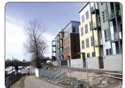
The Midtown Lofts are an example of new residential development on the Midtown Greenway between Bryant and Colfax. New residential development on the Midtown Greenway in Phillips West should be medium to high density, face the Greenway, and have setbacks that allow unobstructed solar access to the Greenway.
