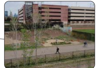
Benches and plantings have enhanced the usability and experience along the greenway. There is strong neighborhood support for expanding amenities and public access to open spaces at the greenway and 5th Ave.
