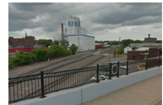
Existing Conditions along Central Avenue
