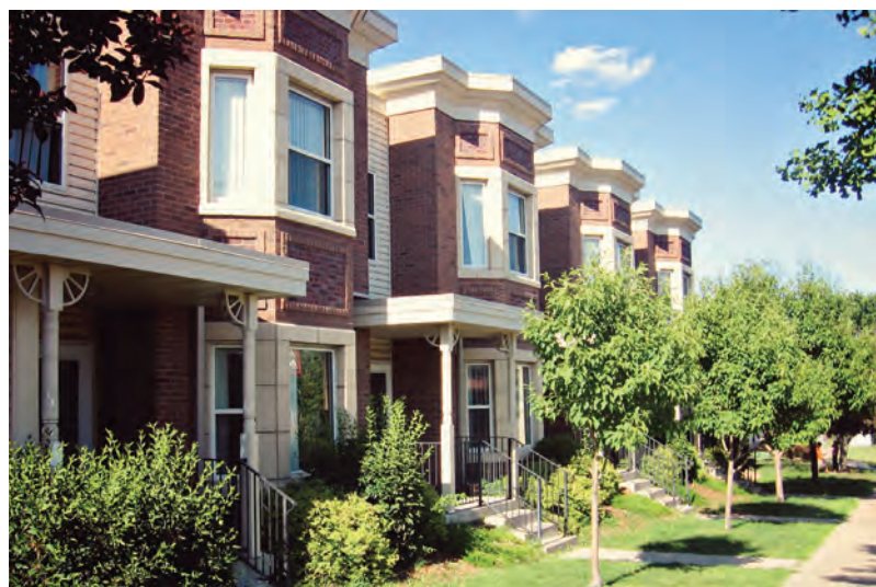
Low density housing: 11 dwelling Units per acre. 3824 44th Street.
