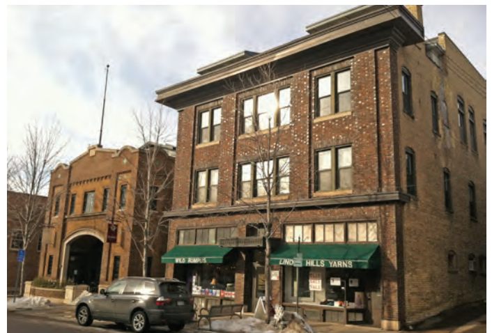
Existing buildings in Linden Hills with stepped back roof top additions that reduce the overall visibility of the additional story.
