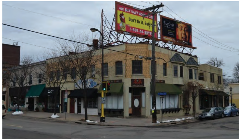
High density housing: 53 dwelling units per acre. 4300 Upton Avenue.
