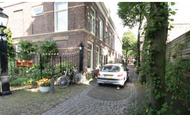
Example of alleyway using rough textured paving and landscaping as traffic calming.
