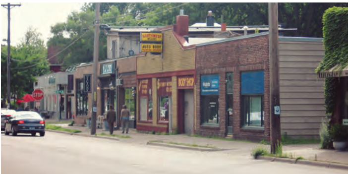
Potential Motor Place Historic District
