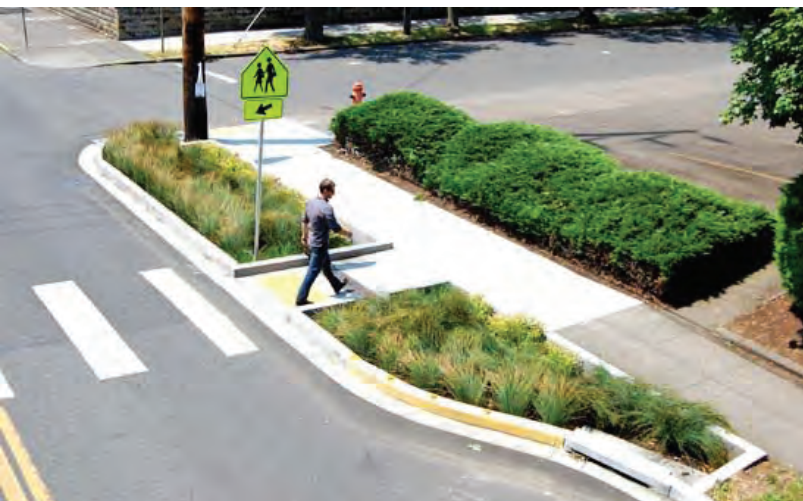
Curb bumpouts can be utilized to provide stormwater benefits.
