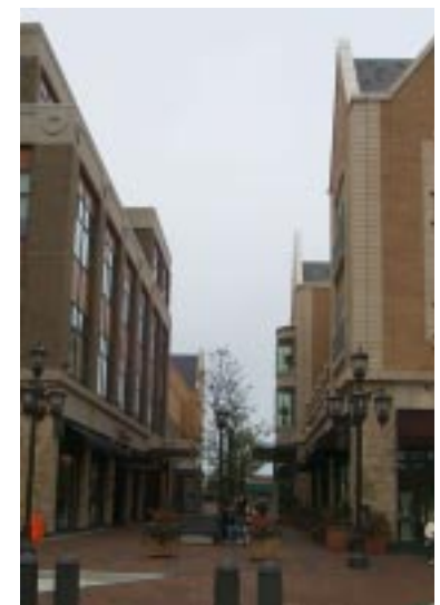
Mixed-use residential and retail oriented towards public plaza with vertical architectural articulation
