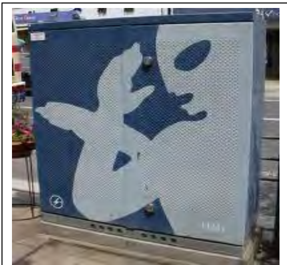
Painted Utility Boxes
