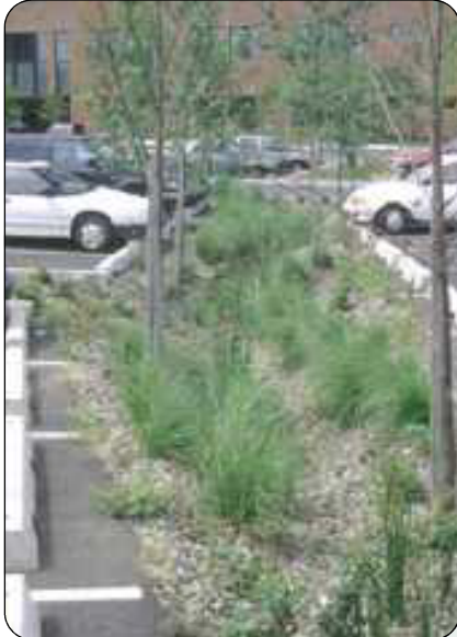
Figure 8.18: This bioswale in a parking lot reduces impervious surface and serves as an alternative filtration system for stormwater run-off.
