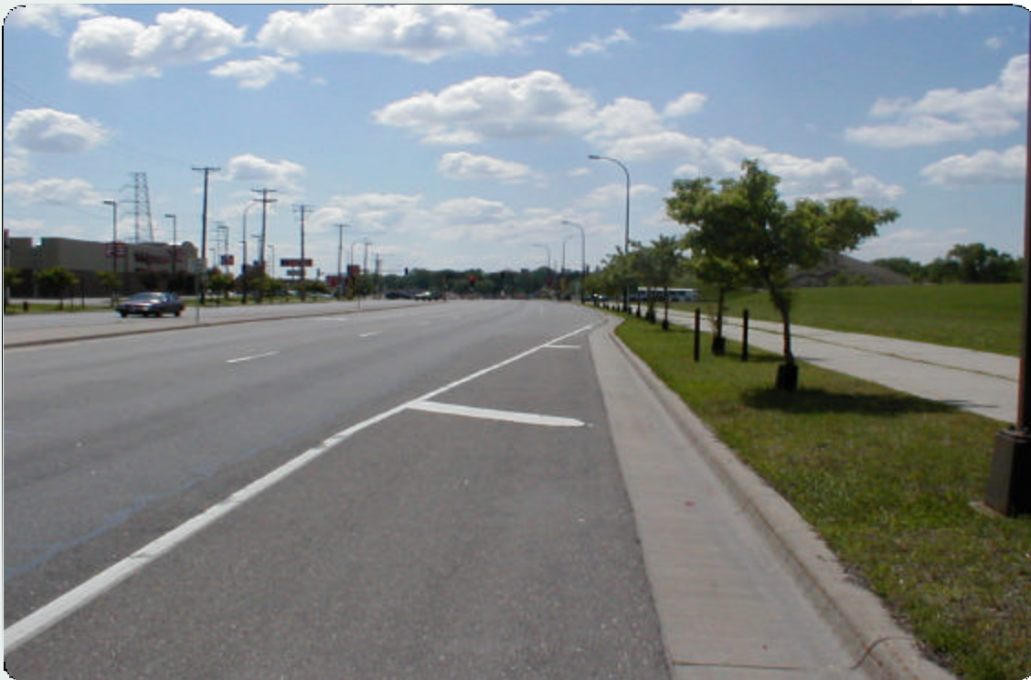
Figure 5.1: Break down lane ("striped" lane) often functions as passing or third travel lane during peak travel times.
