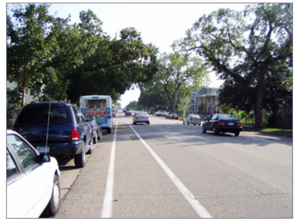
Bicycle lane at Portland Avenue.
