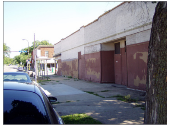
At the intersection of 38th Street and Bloomington Avenue.
