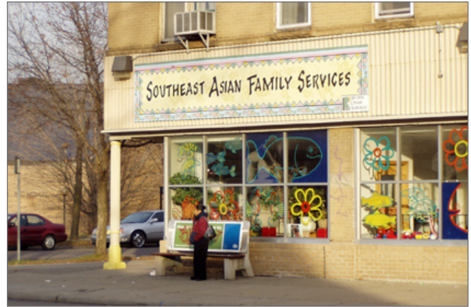
At the intersection of 34th Street and Chicago Avenue, in the Pillsbury Focus Area.
