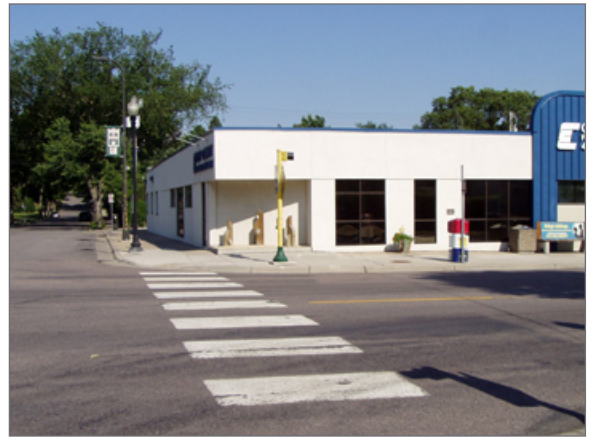
Recommended “zebra” crosswalk markings. Photo: 47th Street and Chicago Avenue.
