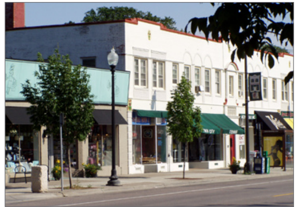
Pedestrian lighting, tree grates, and street furniture at 48th Street and Chicago Avenue.
