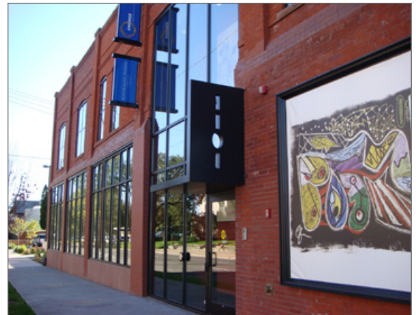
An example of what is possible: the recently rehabilitated building at 1101 Broadway Avenue, in North Minneapolis, now hosts a bank, community development organizations, and a coffee shop.
