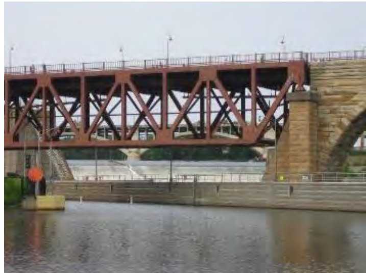
Upper Saint Anthony Falls Dam, upstream of the Stone Arch Bridge
