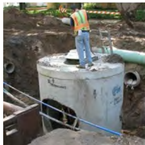
Grit Chamber During Construction
