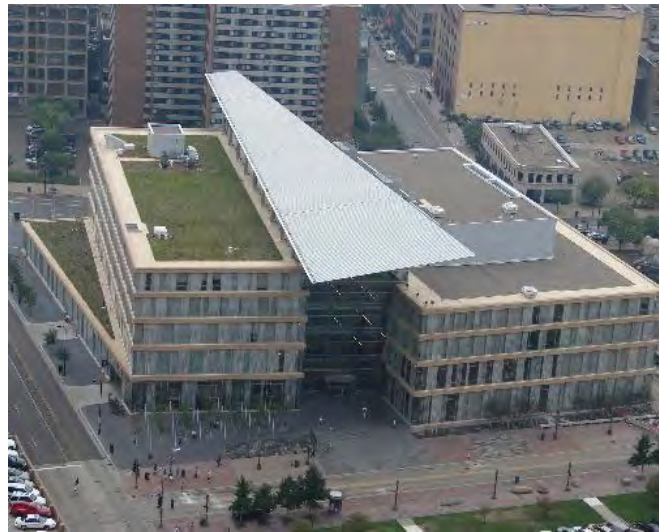
Green Rooftop on Minneapolis Central Library
