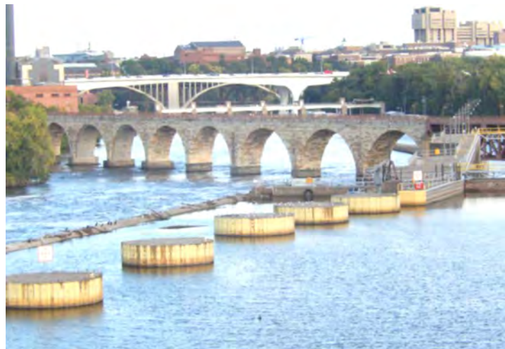
Stone Arch Bridge
