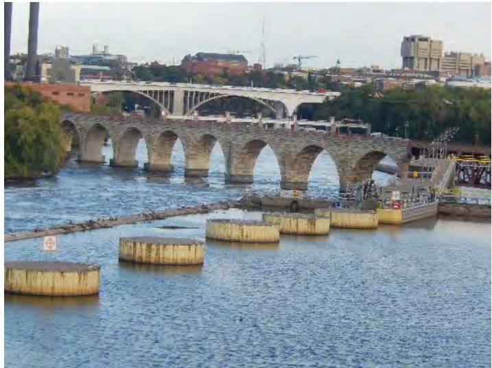
Upper Saint Anthony Falls Lock and Dam, upstream of lock
