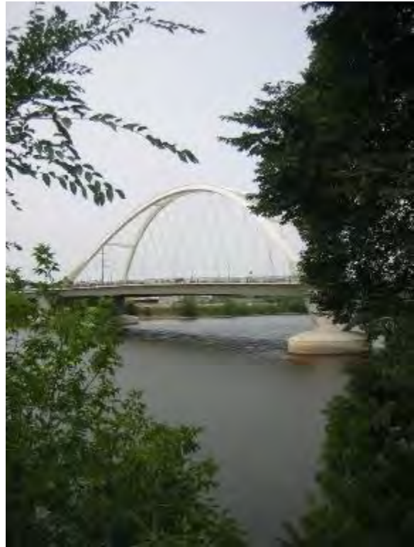
Mississippi River at Lowry Avenue
